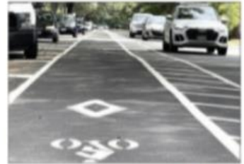
Photo by Carlos Aguilar The City of Houston's "rehab" of Heights Boulevard between 14th and 20th streets included surface milling to improve the ride as well as creating a 3-foot buffer between bicyclists and vehicle traffic.
