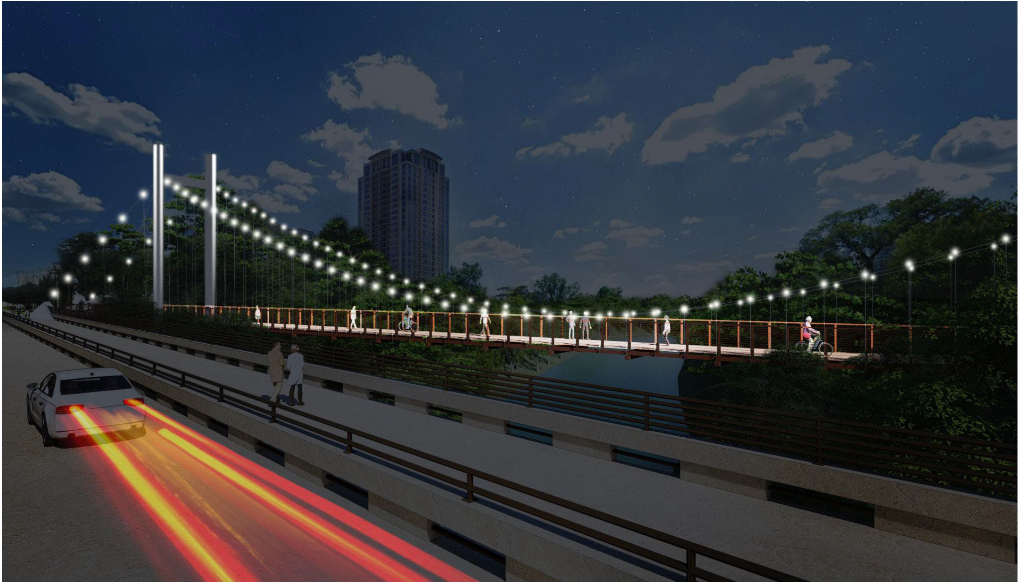
Memorial Park Connector - The Bayou Bridge Houston, Texas
